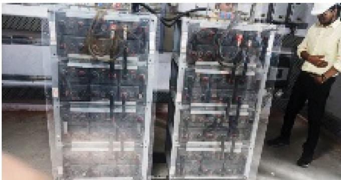
Current renewable microgrids use lead acid batteries, limiting performance and life
